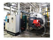
The water content can be quickly transformed into steam. Our boilers always have sufficient steam reserve, even during sudden peak demand period. Using gas, oil or dual fuel burner, the flame intensity is matched virtually instantly to the steam or hot water consumption, taking into account the fuel characteristic.
